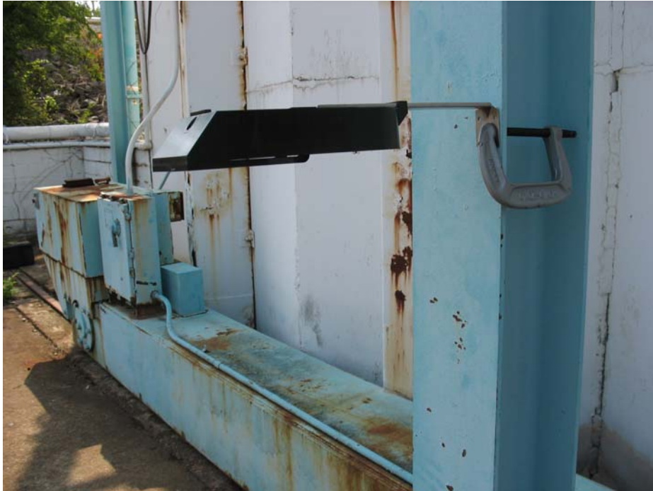
Photograph No. 1 Typical Dry Fire Setup (Initial Design)
